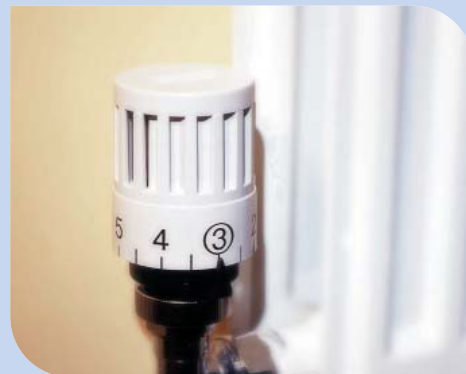
A typical example of a thermostatic radiator valve (TRV) connected to a radiator
