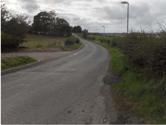
Photograph 1: View looking north/north-east
