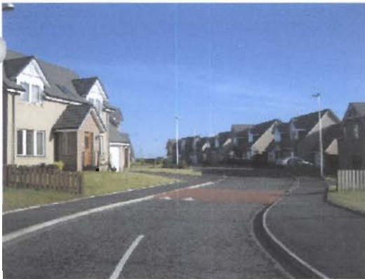
Photograph of recently completed housing to south
