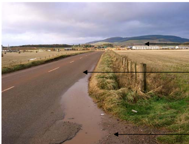
View looking West along B966 road
