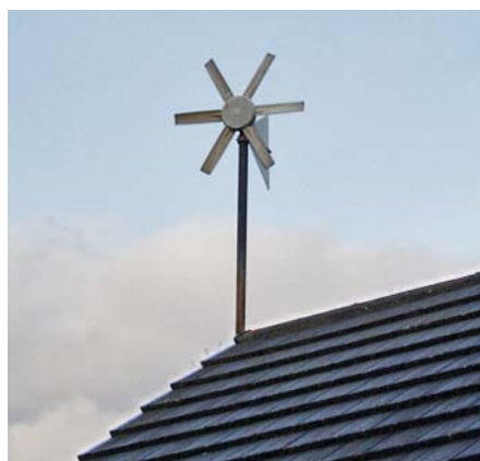
Roof mounted domestic wind turbine
