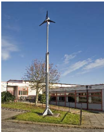
Free standing (non-domestic) wind turbine
