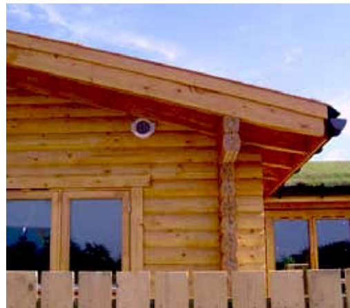
Vent for the air-source heat pump, from of NIBE Industrier, courtesy of Ecoliving Ltd.
