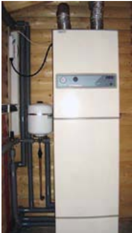
Heat pump system (large - FIGHTER 315P, which replaces both the conventional gas condensing boiler, hot water tank and the separate heat recovery ventilation system) from of NIBE Industrier, courtesy of Ecoliving Ltd.
