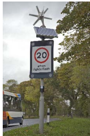
Solar/Wind Turbine speed sign
