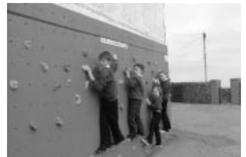
Bracoden Primary School - Panel Fixed
