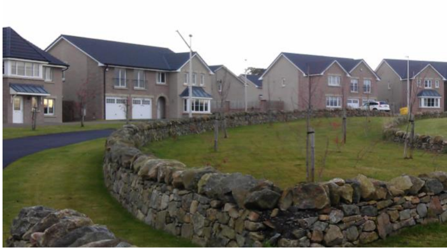
Figure 28: use of drystone dyking
