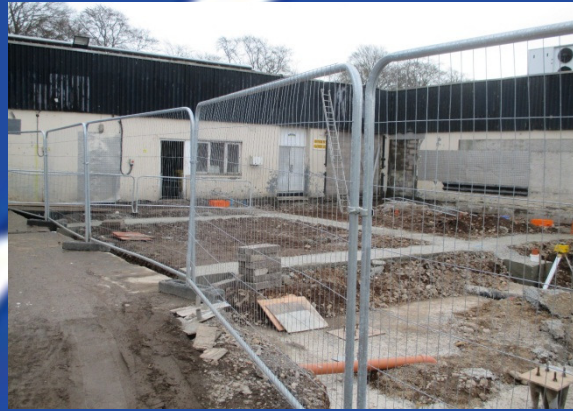
New foundation for Plant room and Dat - Shaub operation
