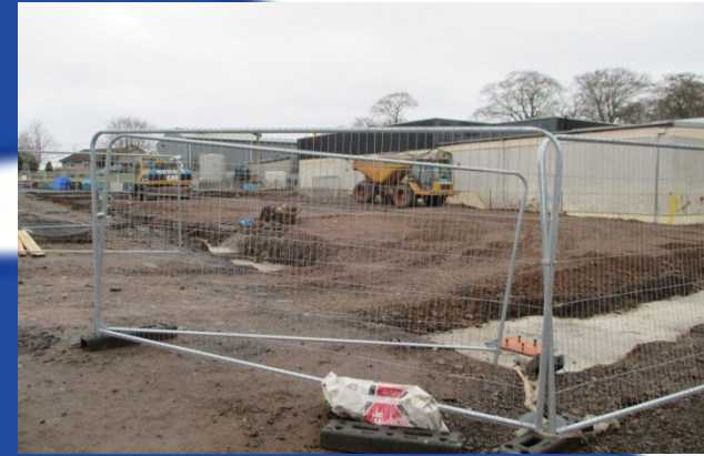
New foundation for Holding Chills and Break / cutting area
