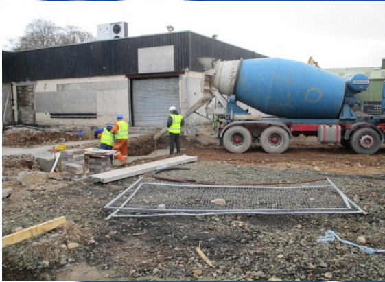
New foundation for Electrical control room
