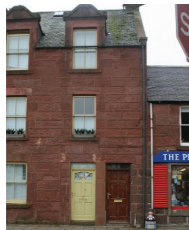
Red ashlar sandstone and pared pointing
