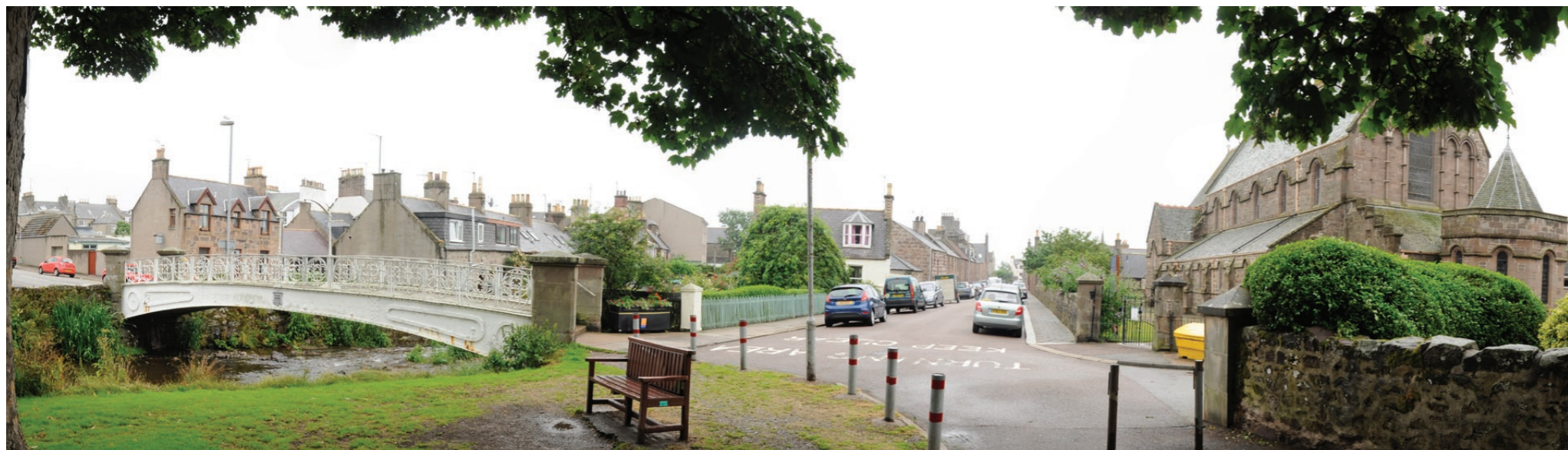
(a) White Bridge
