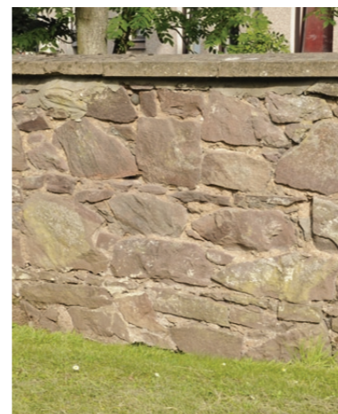
Coursed sandstone rubble wall
