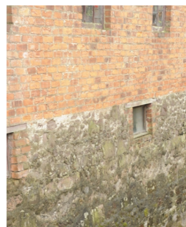
Brick on rubble wall
