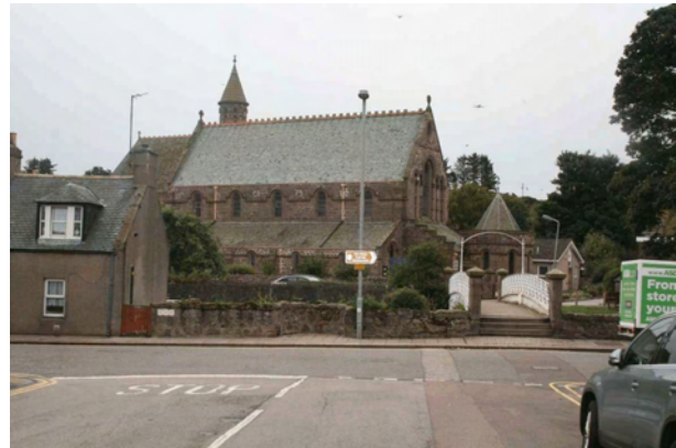
Plate 17 View of the church and White Bridge, looking south
