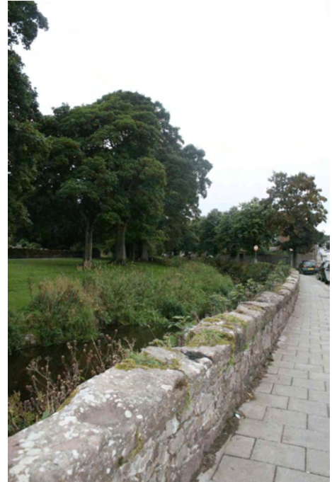
Plate 23 Wall along Cameron Street, looking west
