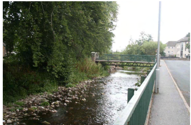
Plate 27 Green Bridge, looking east
