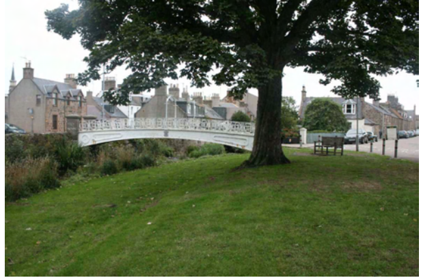
Plate 8 View of the White Bridge, looking east
