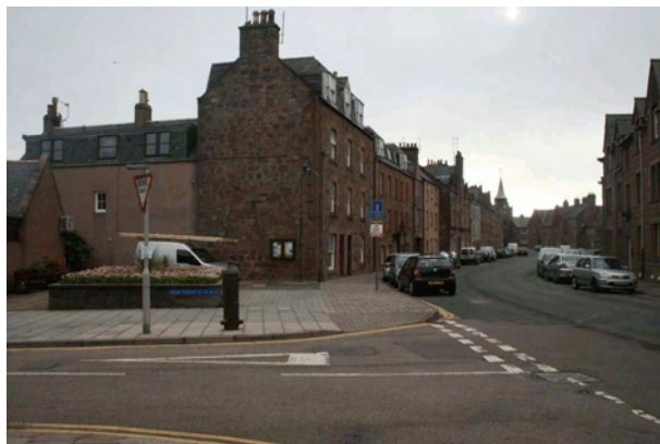
Plate 15 Site of pumping station, High Street
