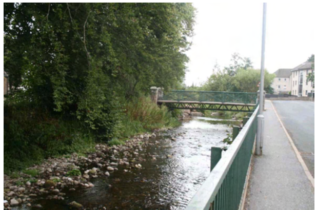
Plate 14 View of the Green Bridge, looking east
