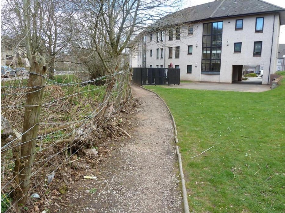
Figure 3-13 Wrack marks on fencing upstream of Woodview Court. (section GLA_179)
