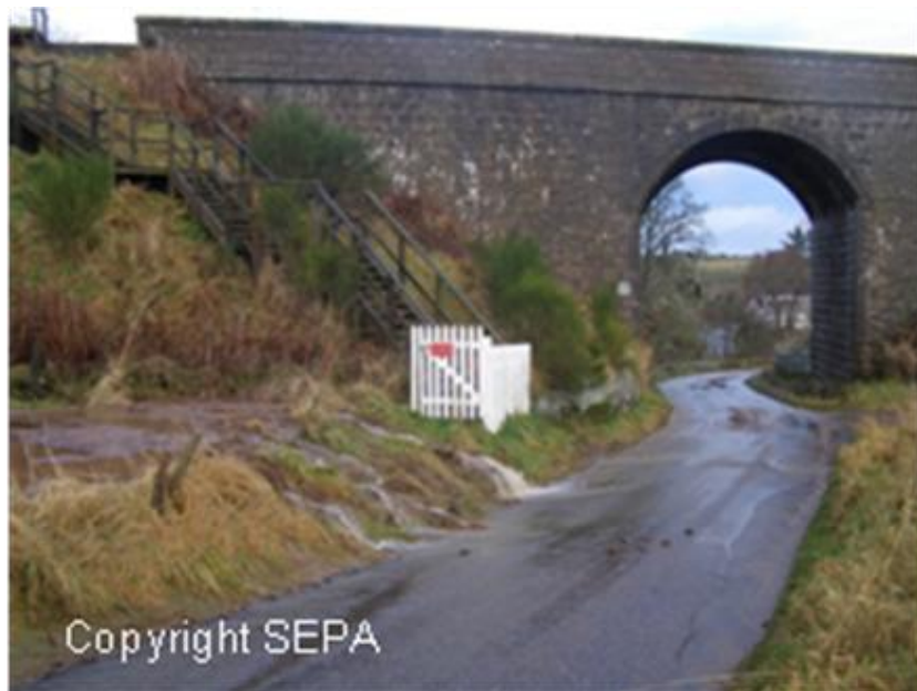
Figure 2-8: Water Flowing off fields upstream of SEPA's Fetteresso gauge
