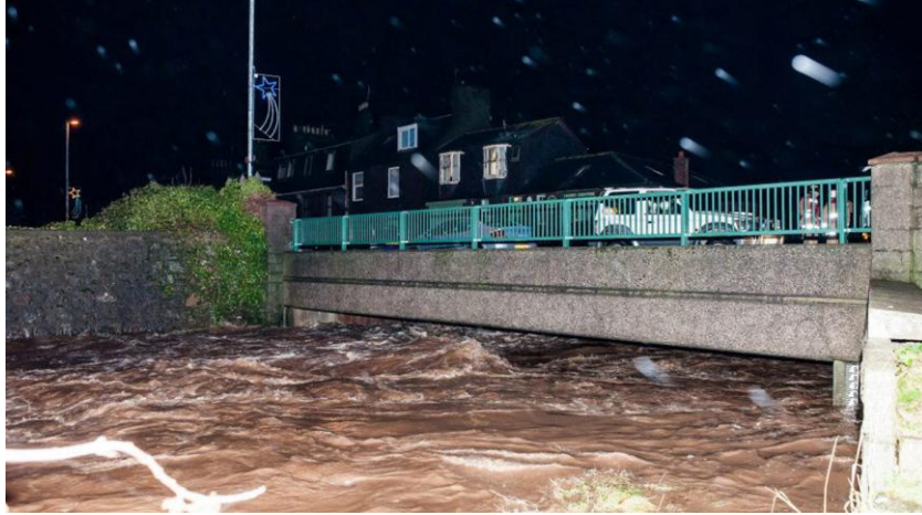
Figure 2-5: River Carron Looking at the Downstream Soffit of Bridgefield Bridge 6
