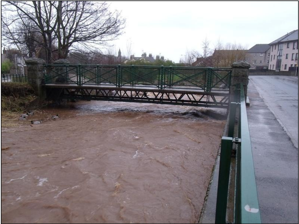
Figure 3-4: Upstream face of Green Bridge taken while sediment bar submerged (Source: Aberdeenshire Council)
