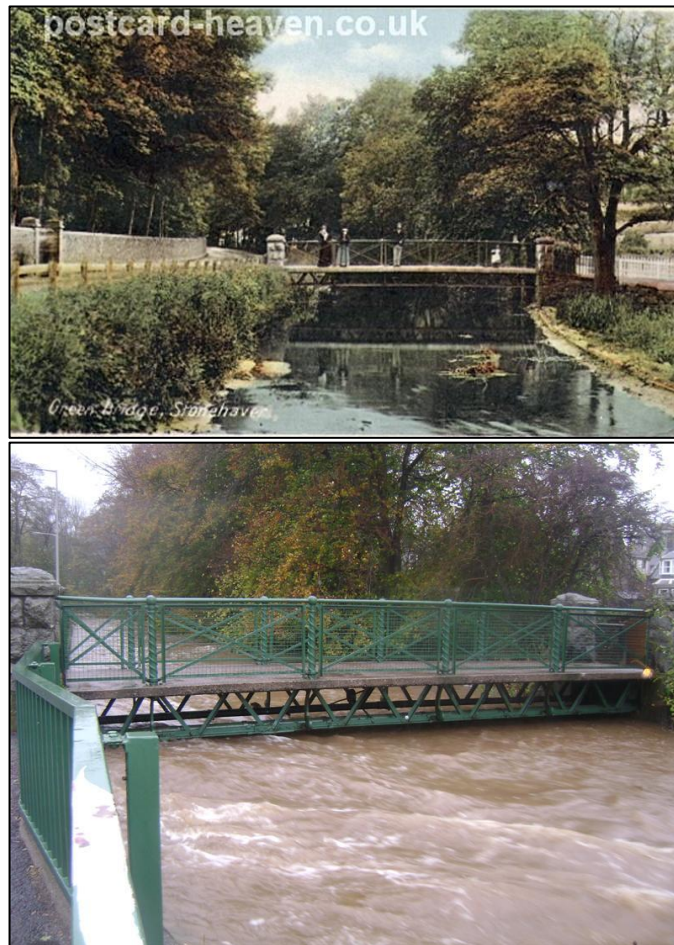
Figure 3-8: The Green Bridge Looking Upstream Prior to Widening of the Low Wood Road and existing elevation (Source: Aberdeenshire Council)
