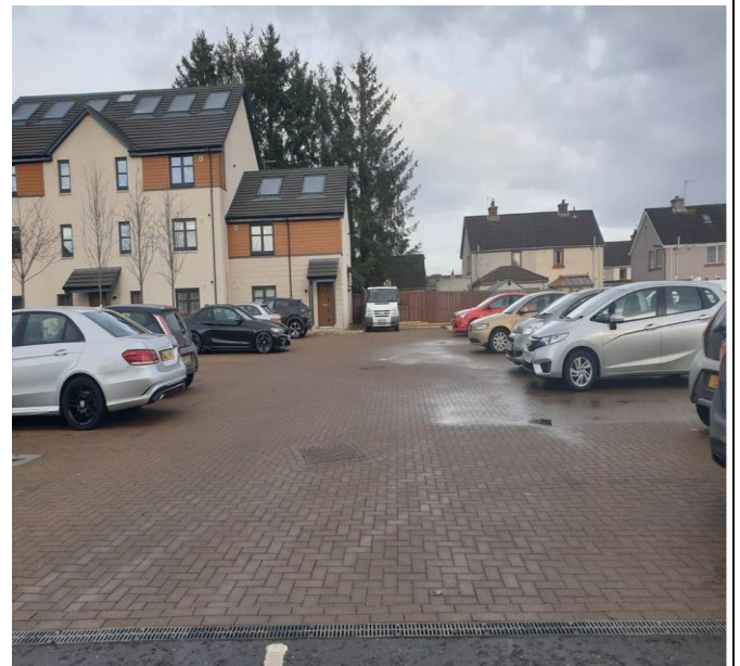
Car Parking Area
