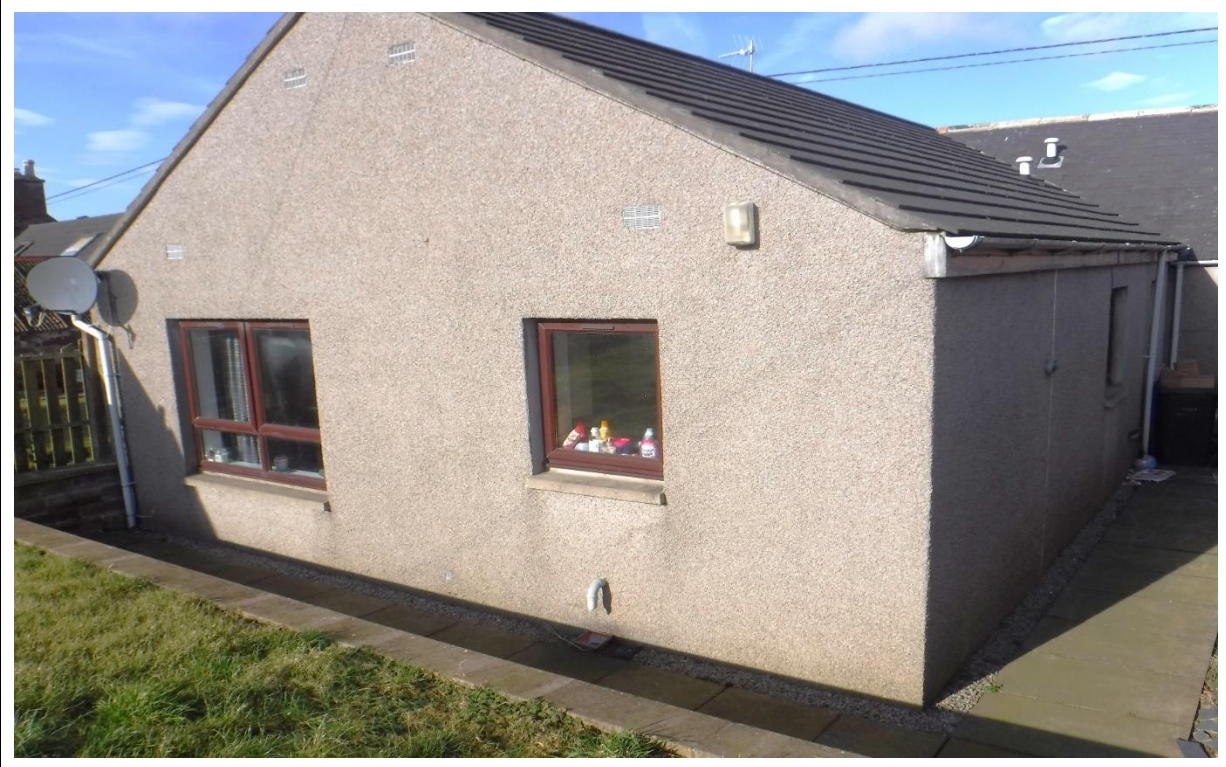
View of Rear of Property
