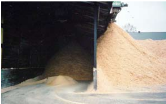
Large scale CHP showing feedstock (Shed)
