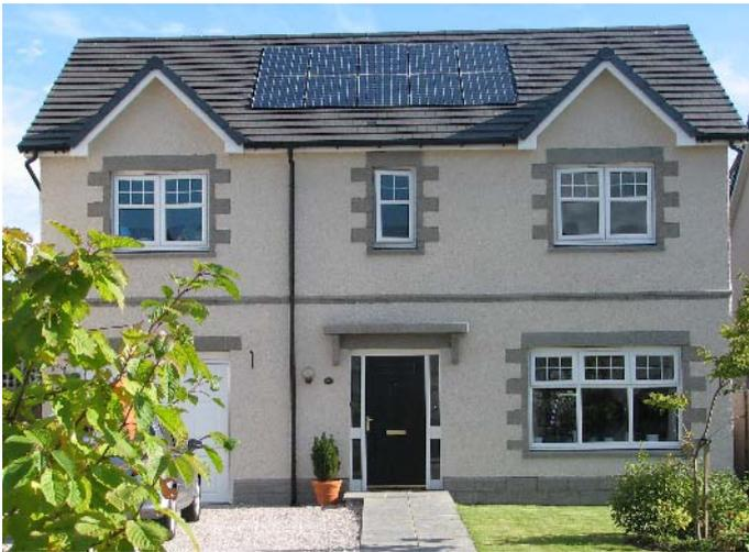
3.60KWp Pitch roof mounted solar pv panels of Aberdeen (image courtesy of AISSC Electrical and Solar)
