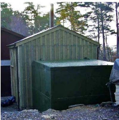
*30kW (heat output) wood fuel system with the green hopper and boiler house attached to main building*
