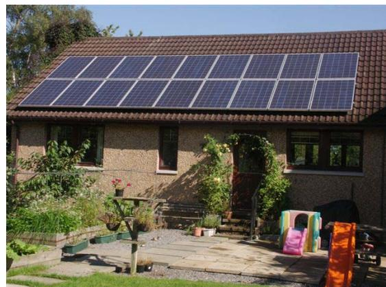
3.87 KWp pitch roof mounted solar pv panels of Aboyne (image courtesy of AISSC Electrical and Solar)
