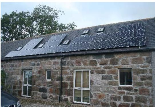
Pitch roof mounted, 3.60Kwp solar pv panels at Drumoak (image courtesy of AISSC Electrical and Solar)
