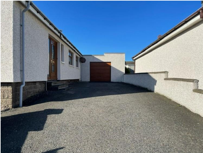
Driveway and Garage
