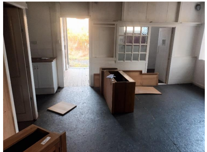
Room 2 Looking Back to Porch
