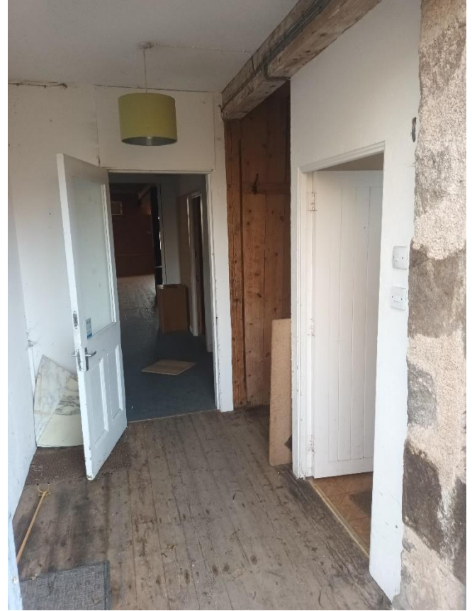
Porch with Toilet Door and Stairwell
